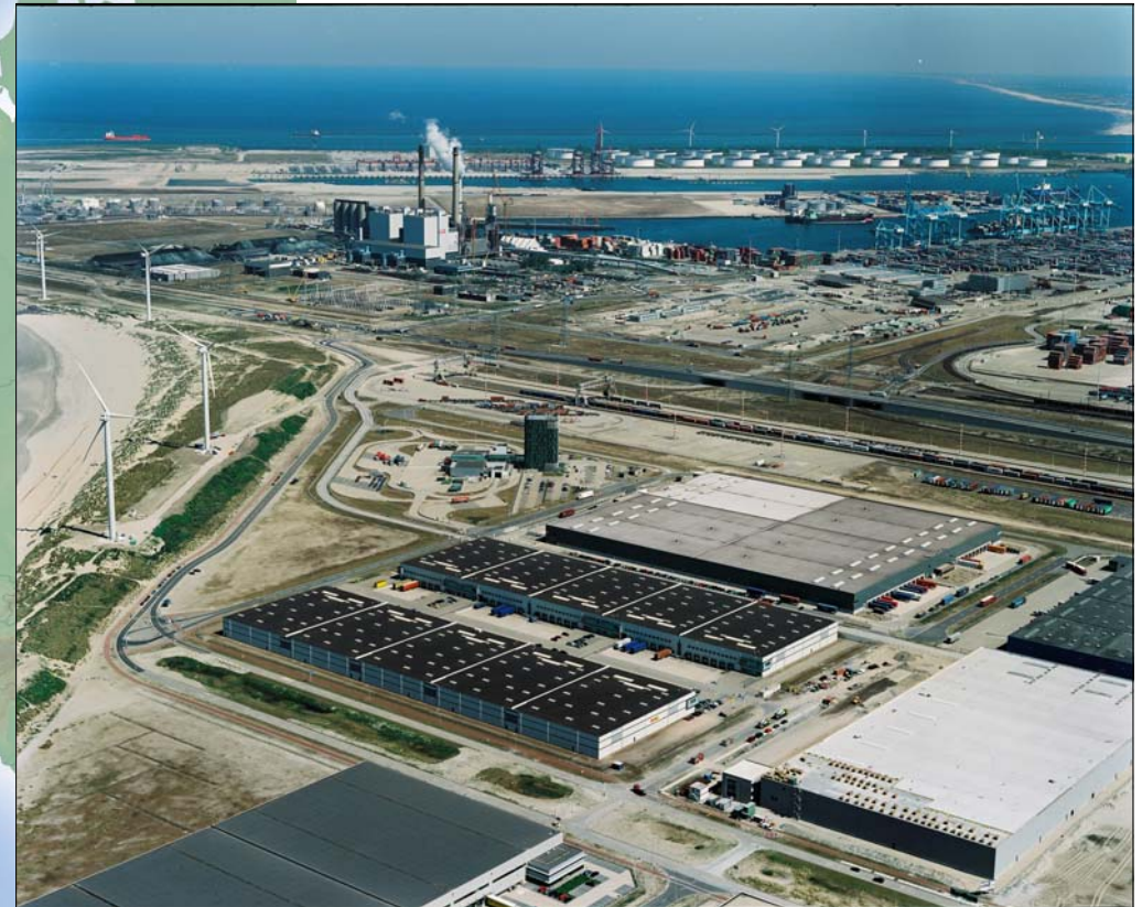
ProLogis Park Maasvlakte, Rotterdam, the Netherlands
