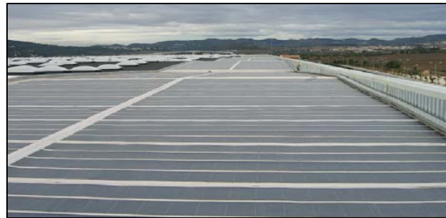
Rooftop solar panels – Spain
